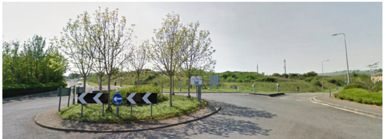
Site Image B: View from Malthouse Avenue of existing highways and Plot 14
