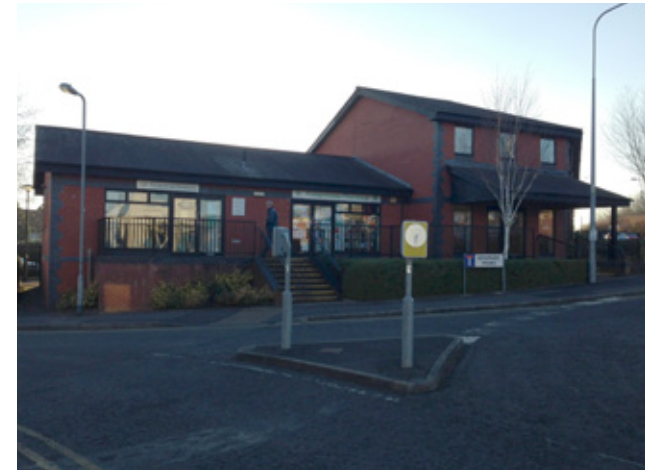
Pontprennau Medical Centre
