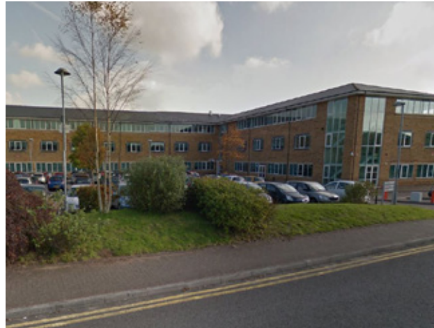
Large office block with surface car park to front
