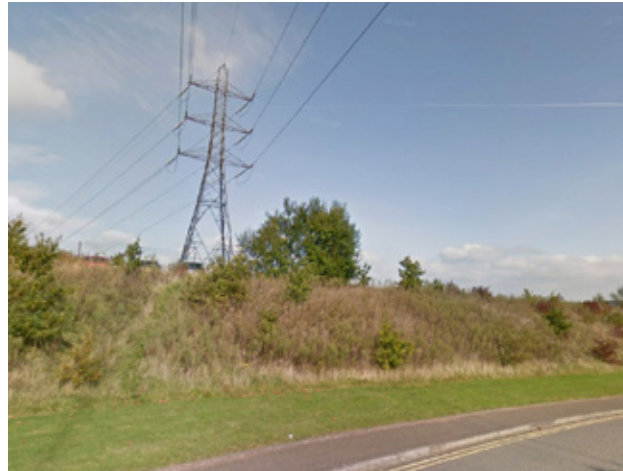
View from Malthouse Avenue of high voltage overhead cables on pylons (near to western boundary of Plot 14)
