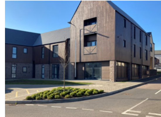
Local precedent: contemporary building with crisp detailing at St Edeyrn's Village Centre.
