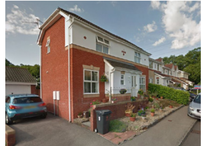
Steps to front entrance in response to topography
